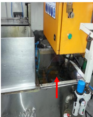
Figure 6: Transparent panel added to the Washing Machine to improve the ease of inspection.
