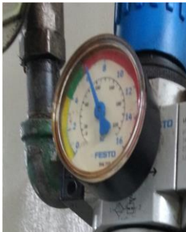
Figure 2: Gauge markings to display acceptable and unacceptable readings.
