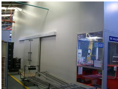
Figure 6: BMC mould area enclosed in order to eliminate contamination to the rest of the area.
